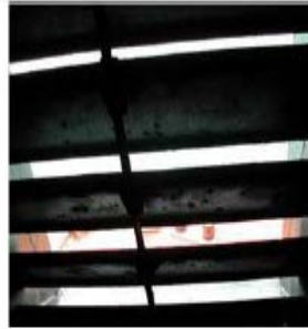
Fire flaps unable to close tight
